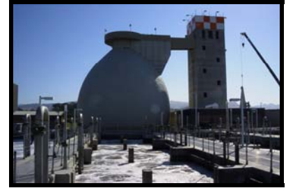
City of Napa Egg Shaped Digester Facility
