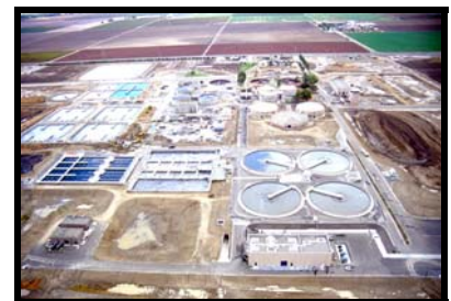
City of Fresno 68 mgd Expansion Construction
