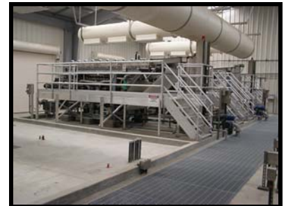
City of Rio Vista Belt Press Dewatering Building
