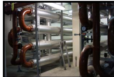
City of NAPA Custom Pipe in Pipe Heat Exchangers
