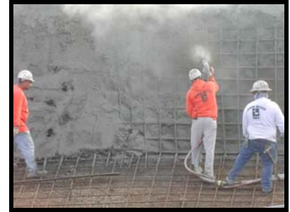
Town of Discovery Bay Oxidation Ditch Construction
