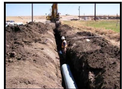
Town of Discovery Bay Export Pipeline Project
