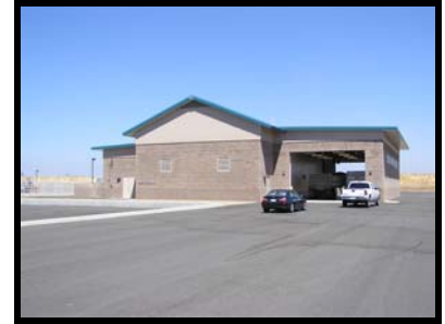
City of Lincoln WWTRF Centrifuge Dewatering Building
