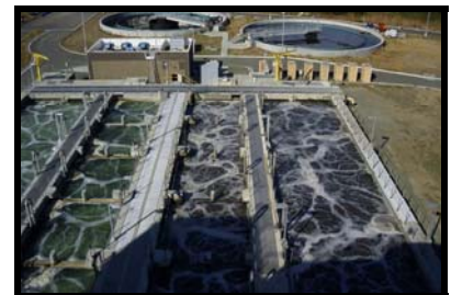
City of Napa 8.5 mgd Aeration System Expansion
