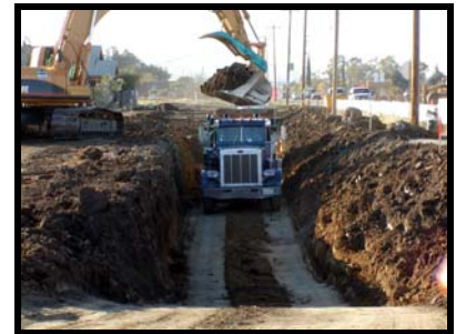
City of Brentwood Lone Tree Way Widening Construction
